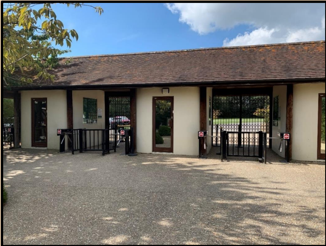
The park side of our entrance gate, showing the metal gate and turnstiles
