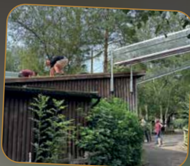
Roof repairs and refurbishment of old loris house for gibbons Tien & Kim
