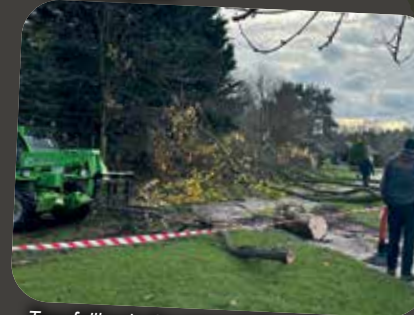
Tree felling in the car park for safety
