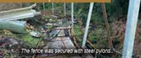
The Capuchin Lodge Fence Repairs
