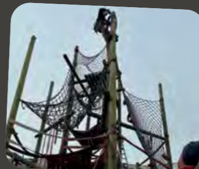
... and we replaced and added some hosing to the climbing frame
