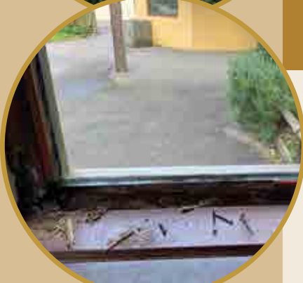
Rotten window frames in former gibbon house
