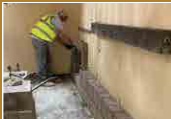
Repairing back wall of Hananya's playroom using additional concrete blocks
